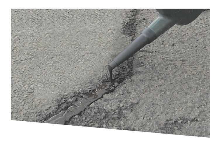
Despite being strong and durable, asphalt will crack over time, even under general wear and tear conditions.
