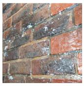
Watco Masonry Waterproofer starts to penetrate the masonry 15 - 20 minutes after application. It will be resistant to light rain after two hours.
