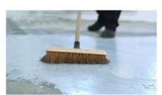
Using a brush or soft broom, spread the primer across the floor. Allow it to soak into the concrete for 15-20 minutes.
