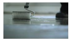
3. Finally, use the spiked roller 3-4 times in different directions to get rid of any air bubbles.
