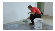
2. Spread Flowtop® across the floor surface with a trowel. It may be convenient to work to a thin batten for depth and edge control but this must be removed before further sections are treated.
