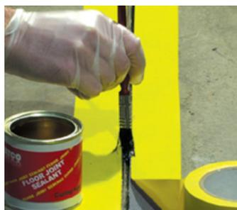
Apply primer by brush to the sides of the joint and allow to dry (approximately 30 minutes at 20°C). Masking tape may be used.
