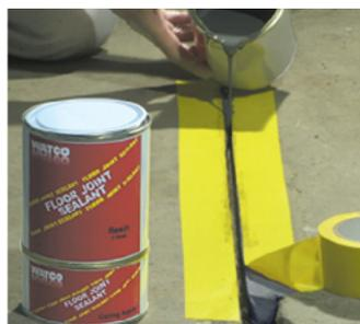
Crimp the rim of the tin to facilitate pouring and pour evenly into the prepared joint, leaving the top of the joint sealant just below the surface of the floor.
